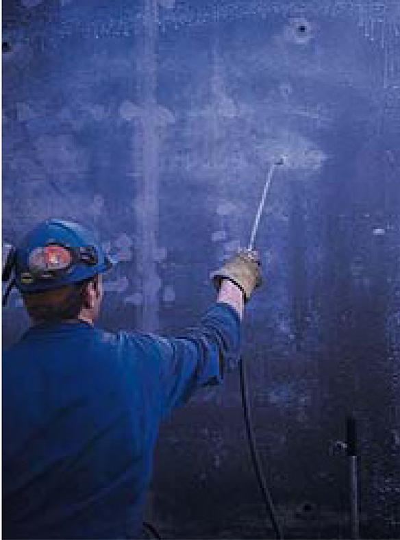
**BIOREL™** should be finely and evenly spread onto the formwork. 1 Liter of **BIOREL™** should cover at least 20 to 30 m<sup>2</sup> of formwork.
